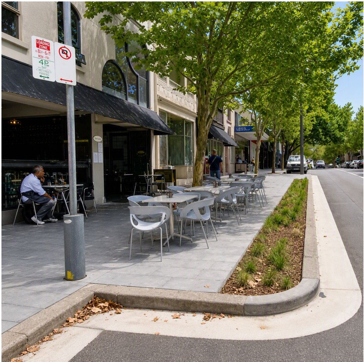
Figure 3. Example of completed footpath extension
